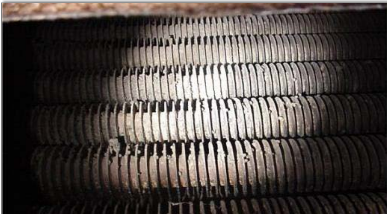
Top view of finned economizer tubes
