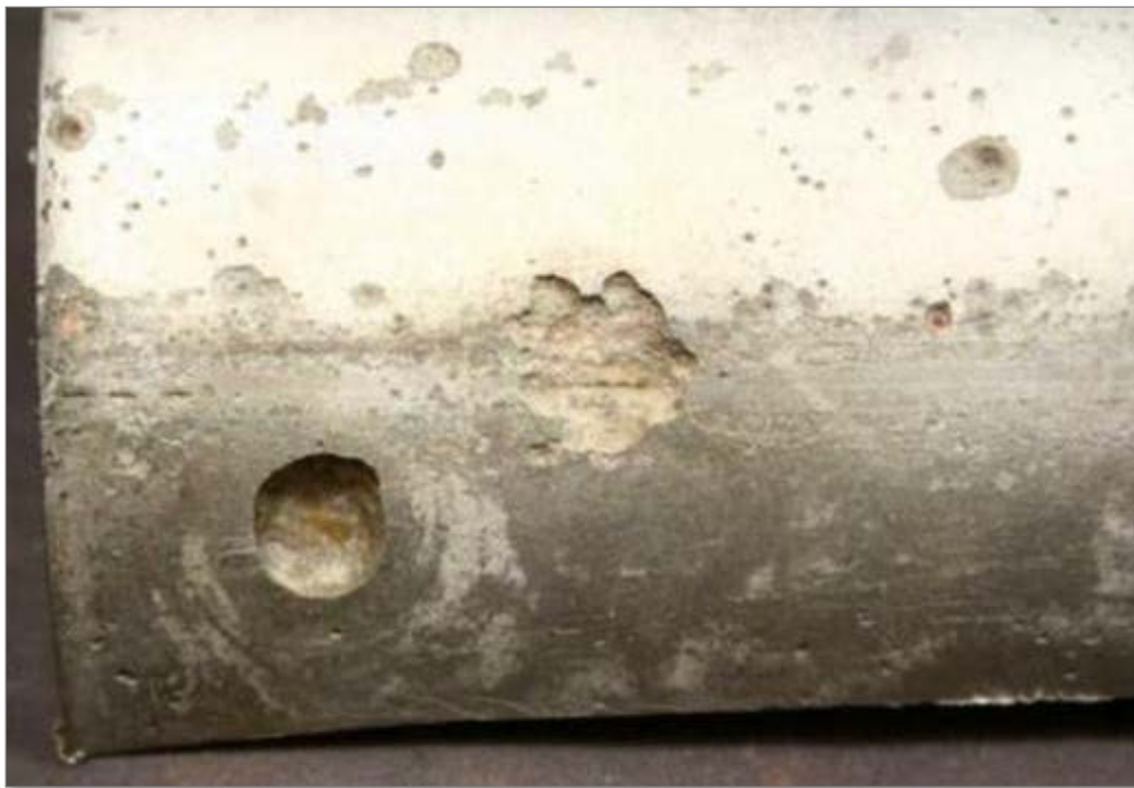
Oxygen pitting, after cleaning
