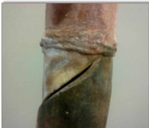
Crack initiation at radial weld
