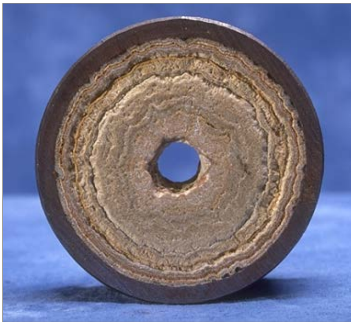
Feedwater line deposits due to years of repetitive hardness intrusion
