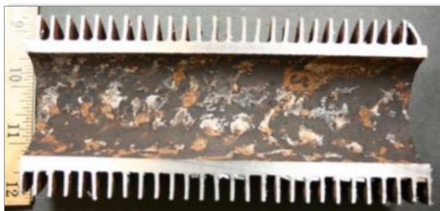
Internal surface of finned SH tube showing deposits from boiler water carryover
