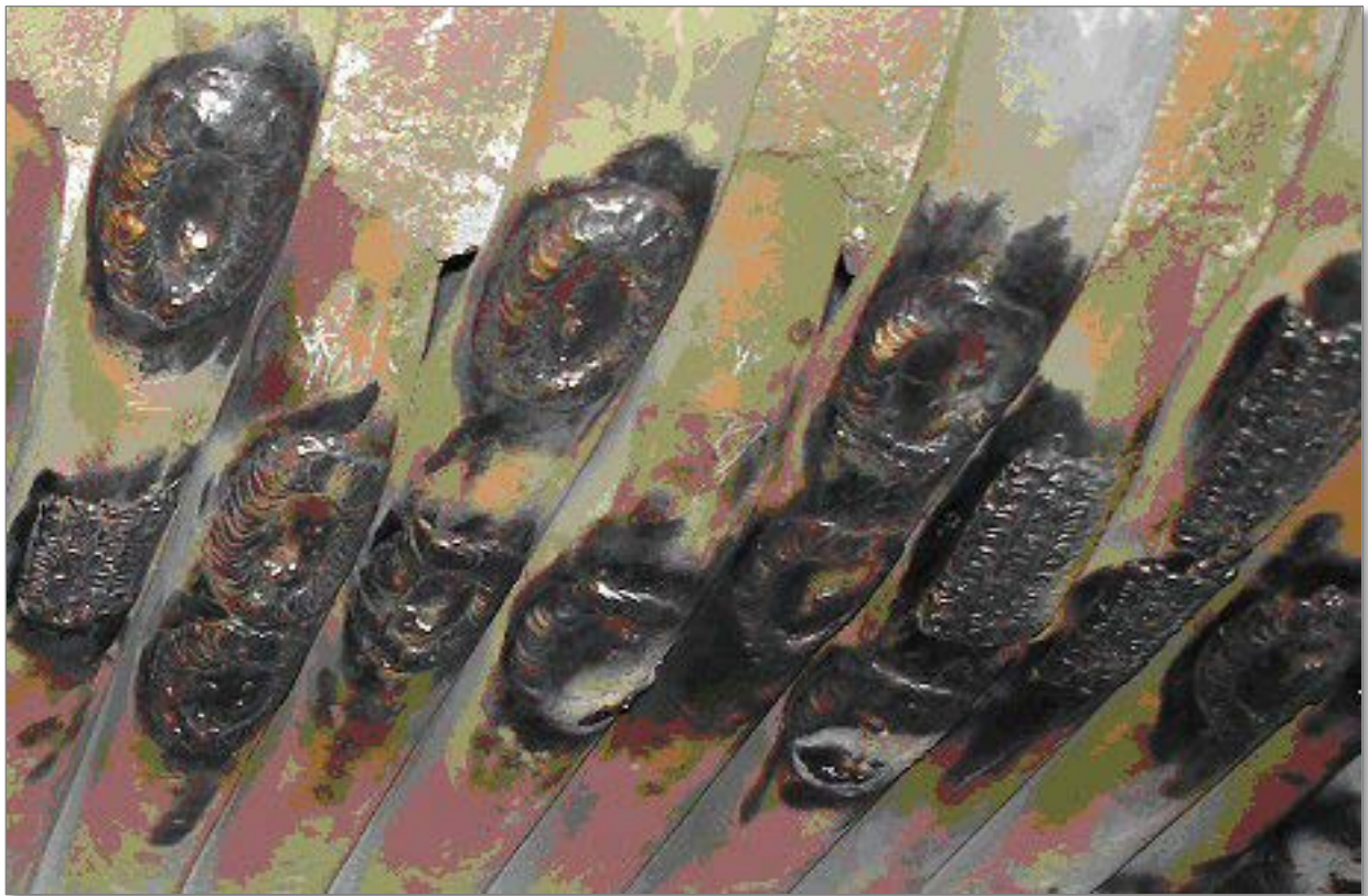
Weld overlay to repair furnace tube bulges resulting from flame impingement
