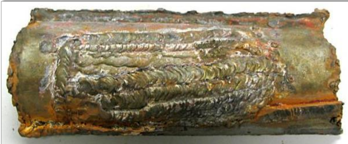
Heavy weld overlay to repair a tube leak
