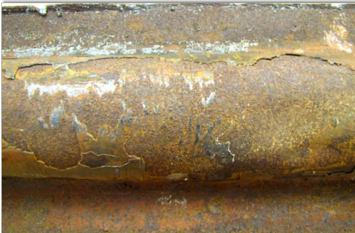
Tube surface metal exfoliation due to flame impingement, overheating
