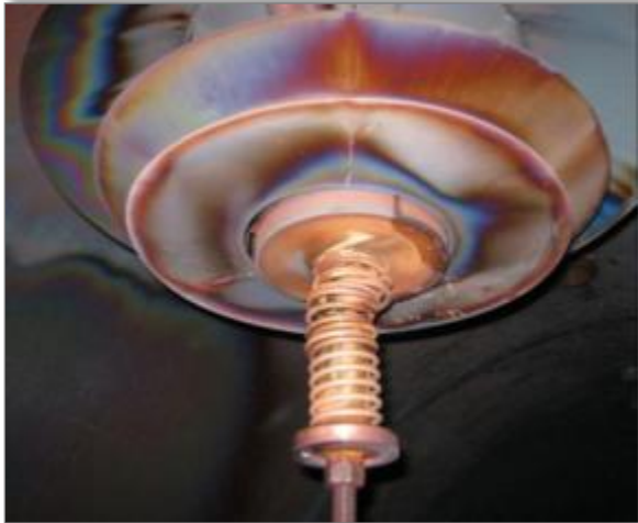
Deaerator spray valve spring failure
