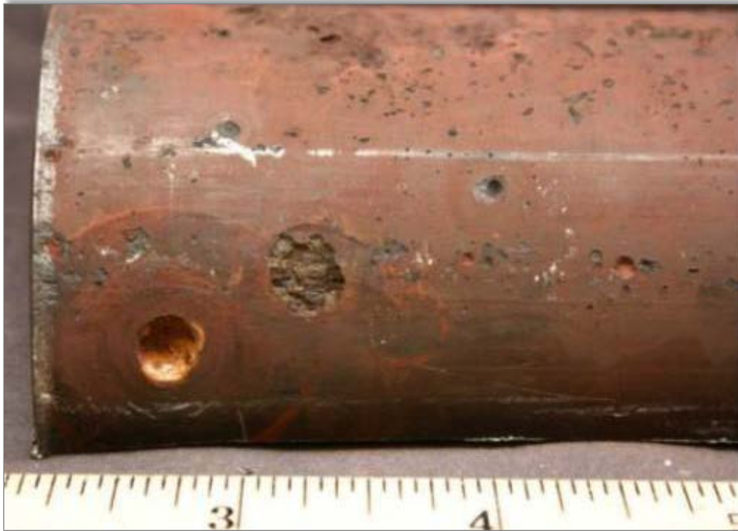
Oxygen pitting, before cleaning
