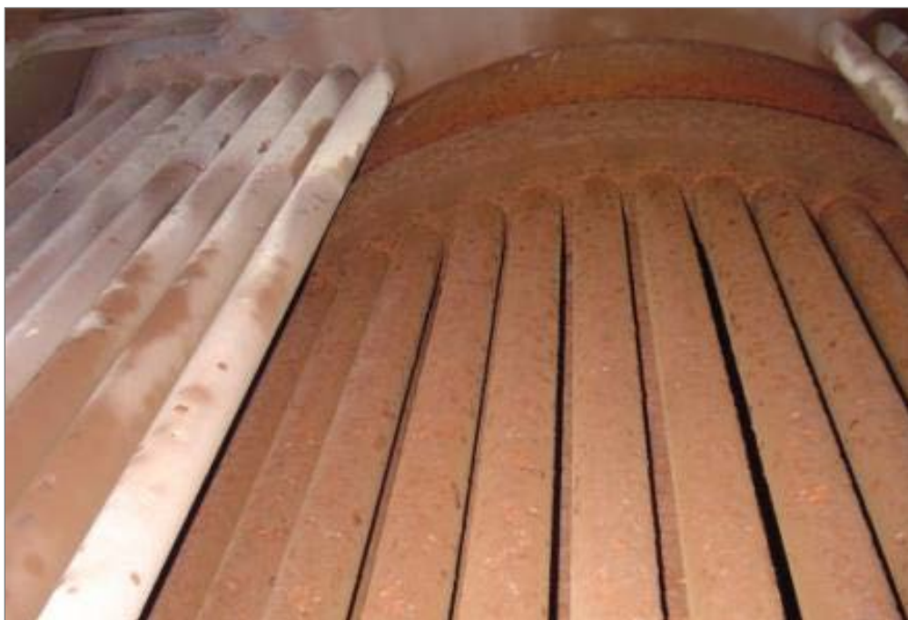
Tubes viewed from man-way, white deposits from evaporation to dryness
