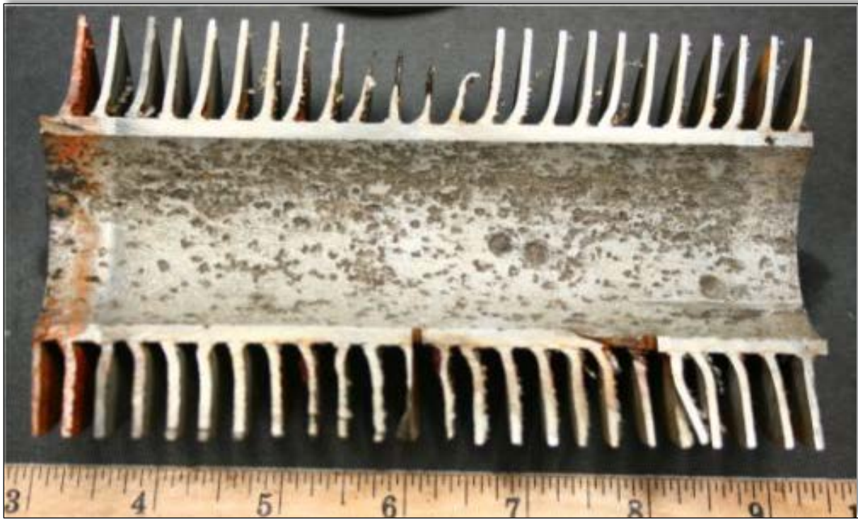
Tube section, cleaned in dilute inhibited hydrochloric acid Oxygen pitting evident after cleaning
